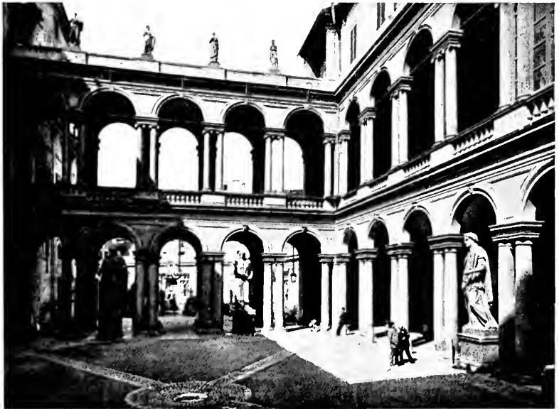
CORTILE OF THE PALAZZO BORGHESE, ROME.
